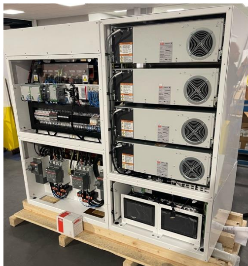
SP300 400kVA. 2x Rectifiers and 2x Inverters
